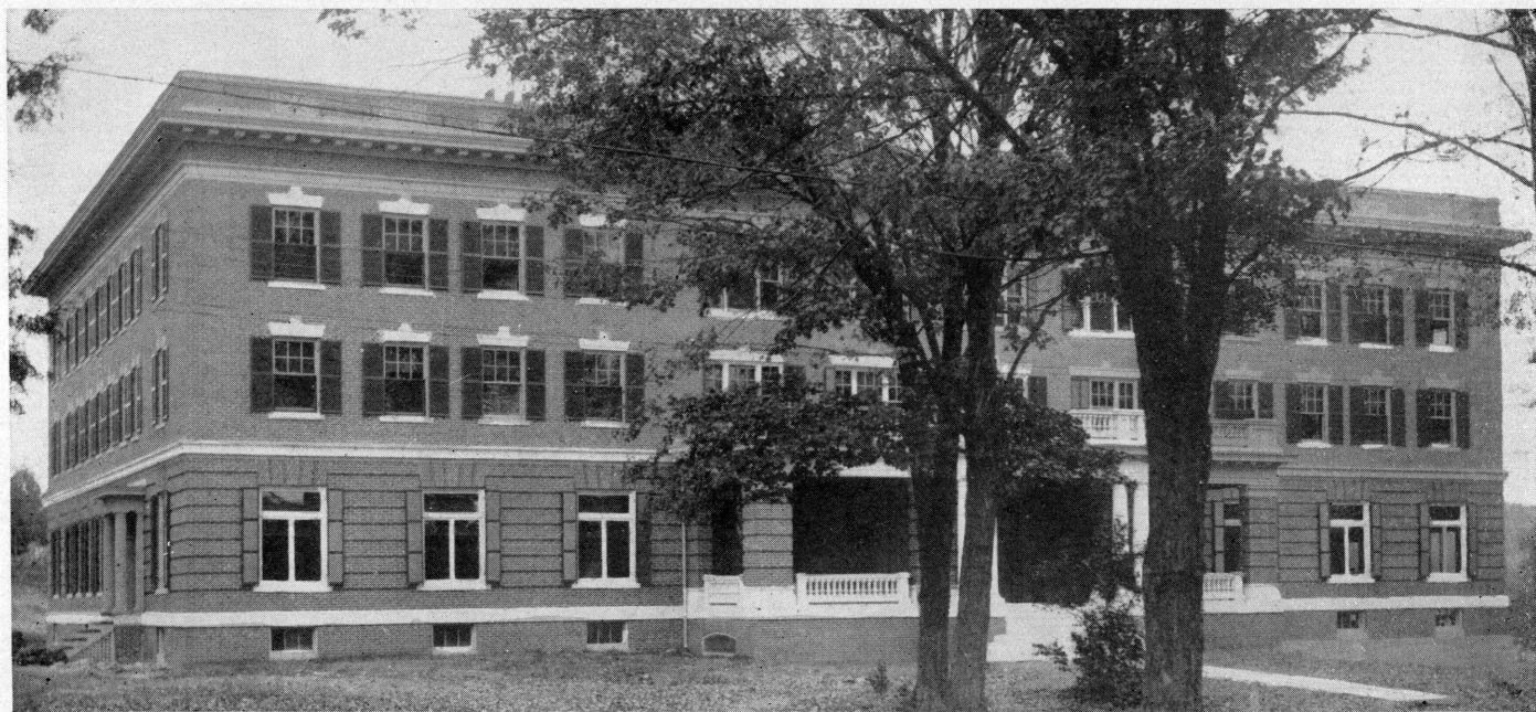
State Normal School, Farmington Purington Hall. Erected 1914
