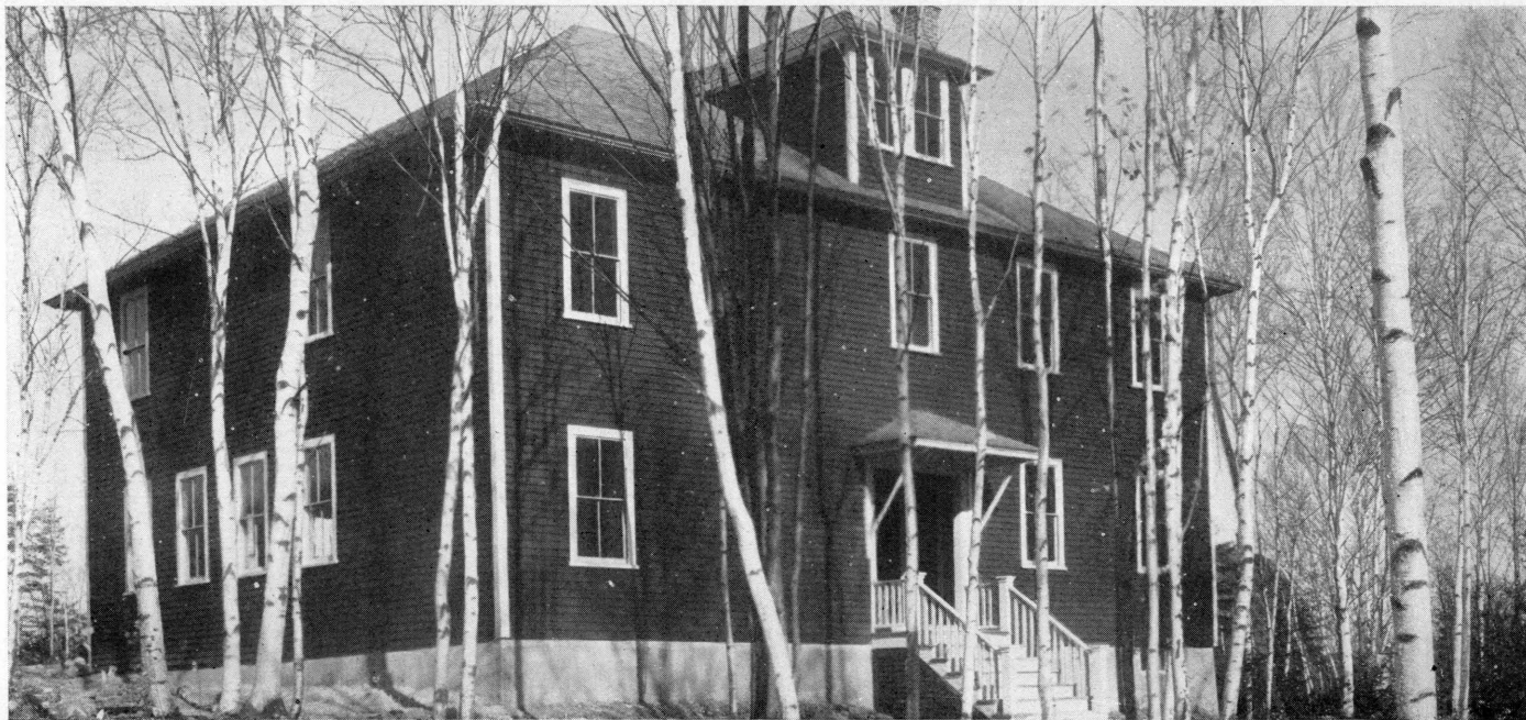
Rockwood—Kineo Station Unorganized Township School. Erected 1914
