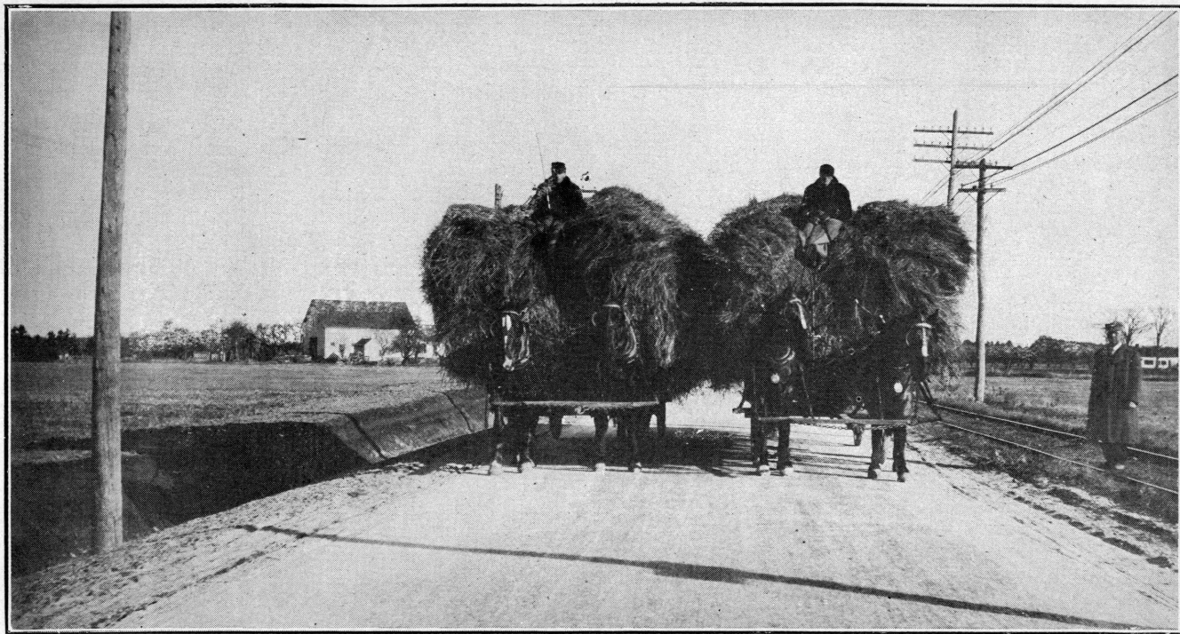
Federal Aid Road. Bituminous macadam surface, showing two loads of hay on a width of 16 feet.
