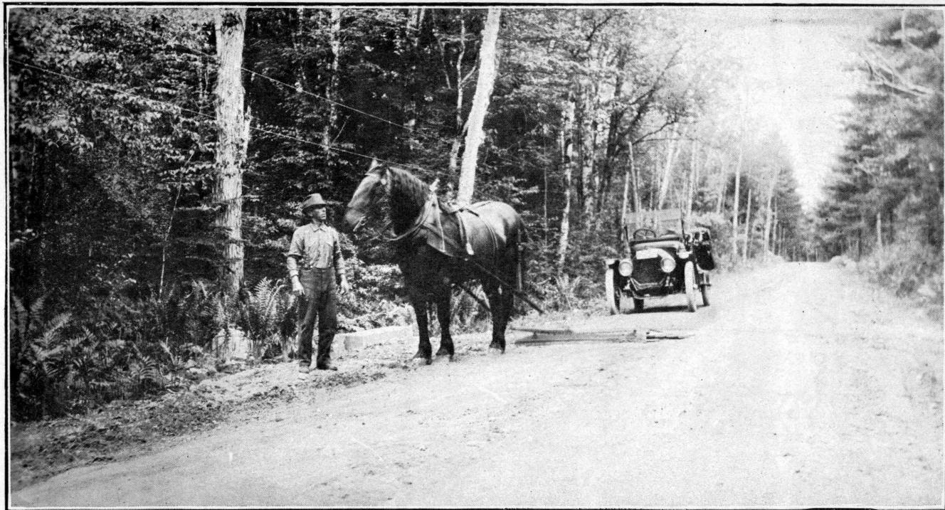
Fryeburg. Patrolman with single horse drag, filling ruts and dragging the loose material from the shoulders toward the center of the road.
