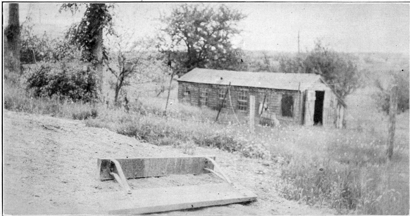
Road Drag used by patrolmen on maintenance of gravel roads.
