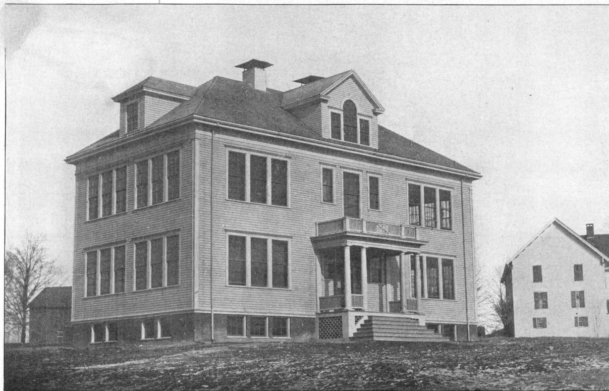
Consolidated School, Grade Building, Buxton, Erected 1912
