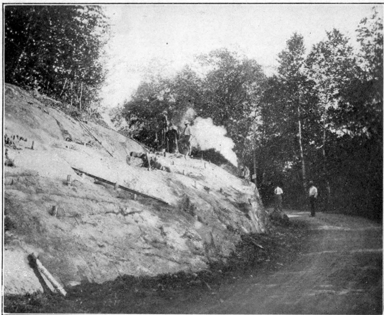
Ledge Excavation. Bingham and The Forks. Before Improvement.
