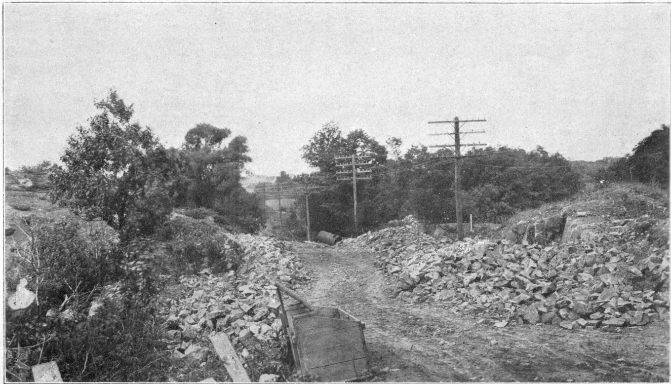
Trunk Line State Road. Grading. York Wells Section.
