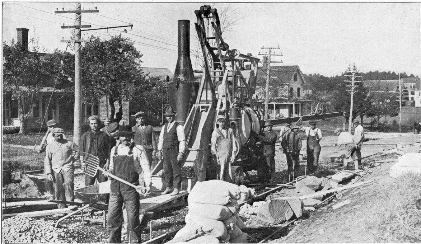
Trunk Line State Road. Laying Concrete. York Wells Section.
