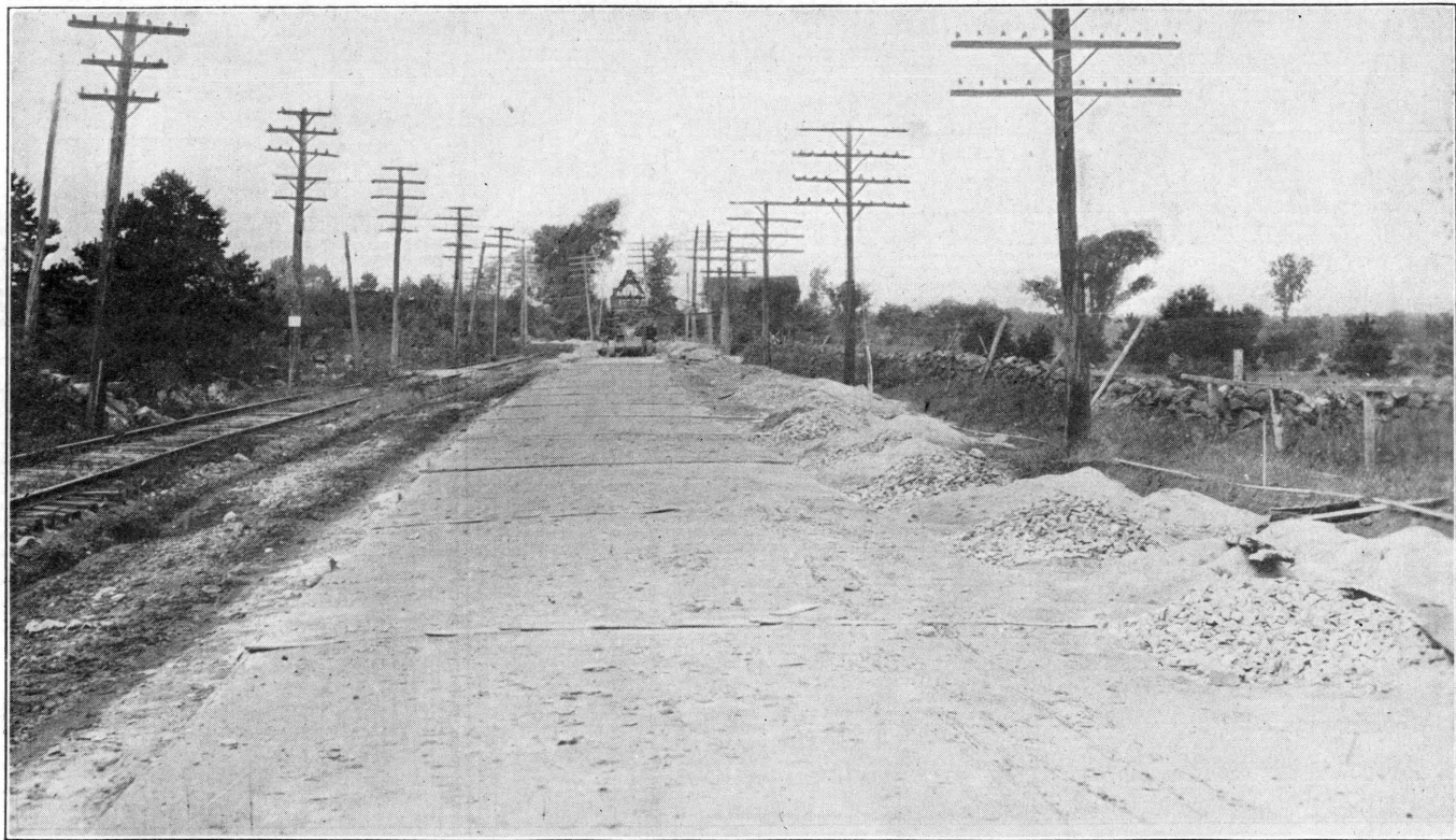
Trunk Line State Road. Wells Section No. 1. Concrete.
