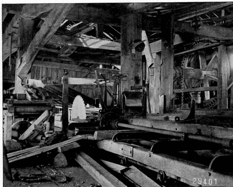
View inside one of the old tide mills still running. Shows rotary saw and carriage (modern) old windlass wheel for hauling logs out of the water; and edger.
