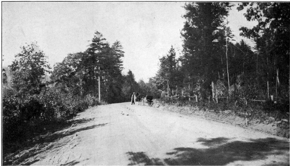
Skowhegan. Section of 1911 State Road. Sand-clay.
