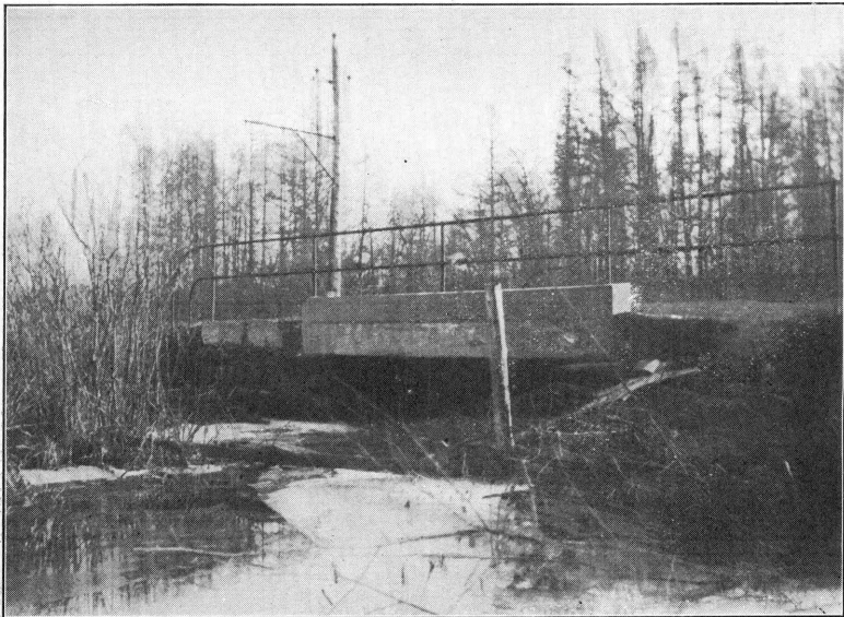
Vassalboro. Reinforced Concrete Bridge. 1911.
