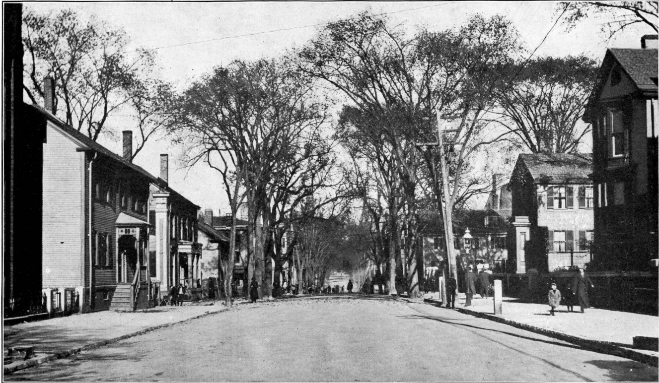
Portland. Section of State Road on Cumberland Avenue after laying concrete pavement.
