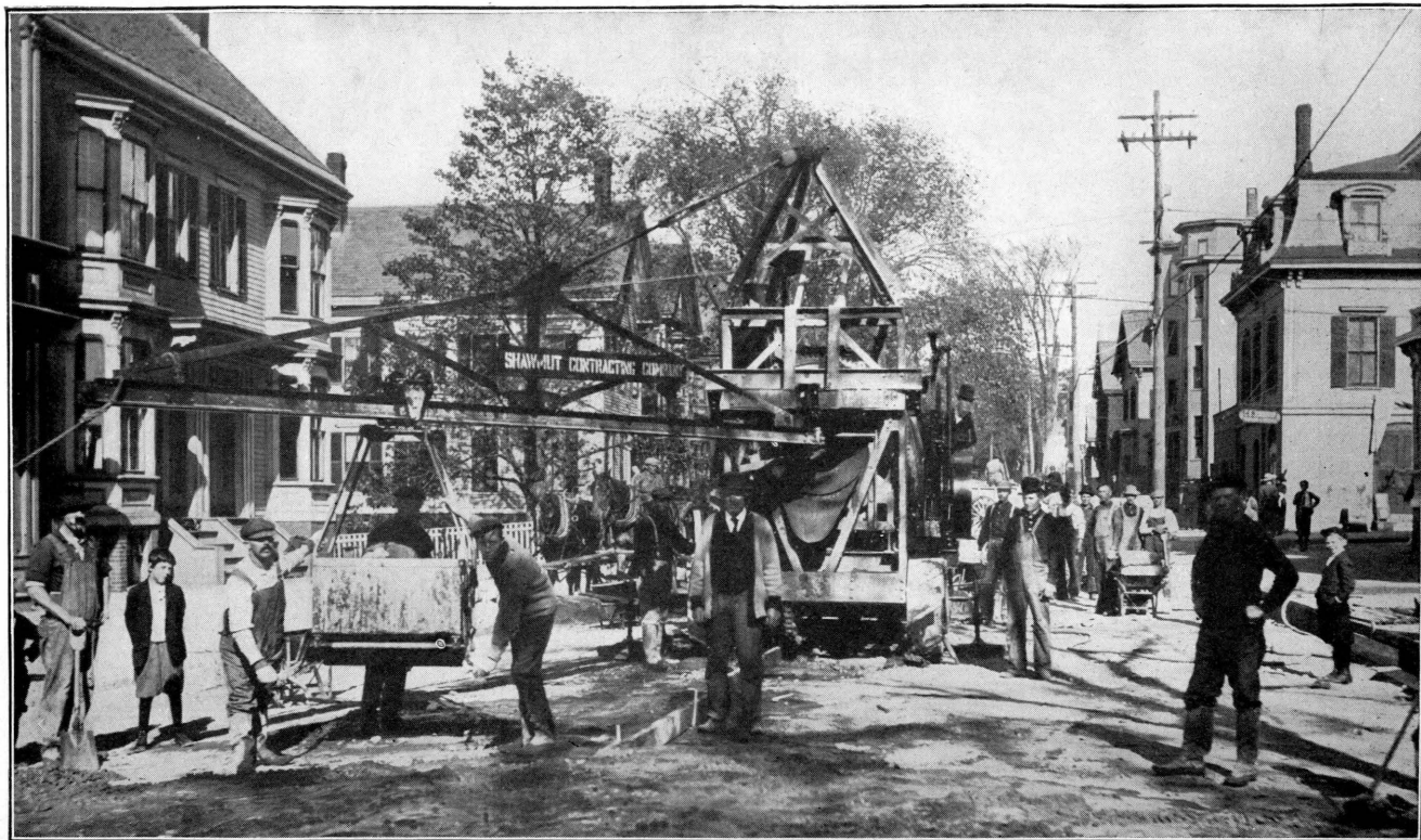
Portland. State Road Work, 1911. Showing method of laying concrete pavement.
