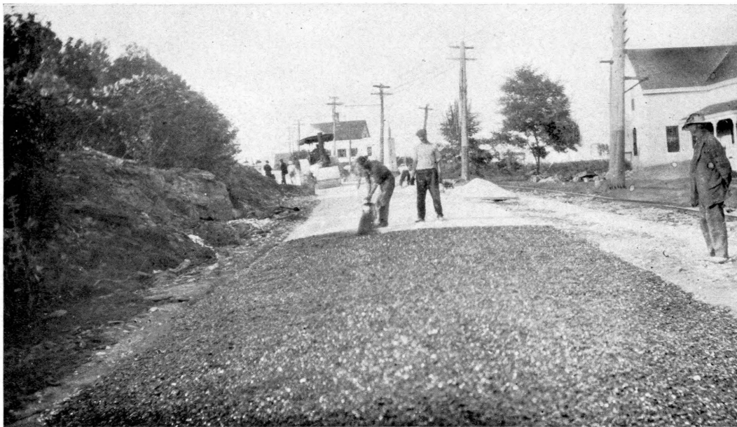
Rockland-Rockport. Trunk Line, showing method of applying bituminous material
