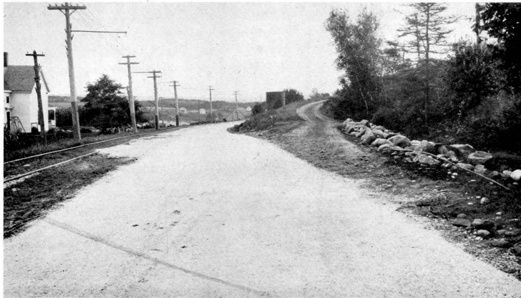
Rockland-Rockport. Trunk Line. Finished section built in 1910. Bituminous Macadam
