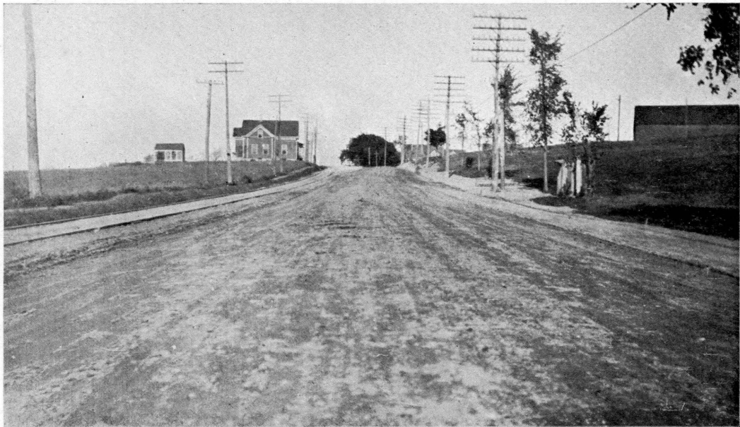
South Portland. Section of Trunk Line, showing road after improvement Gravel surface
