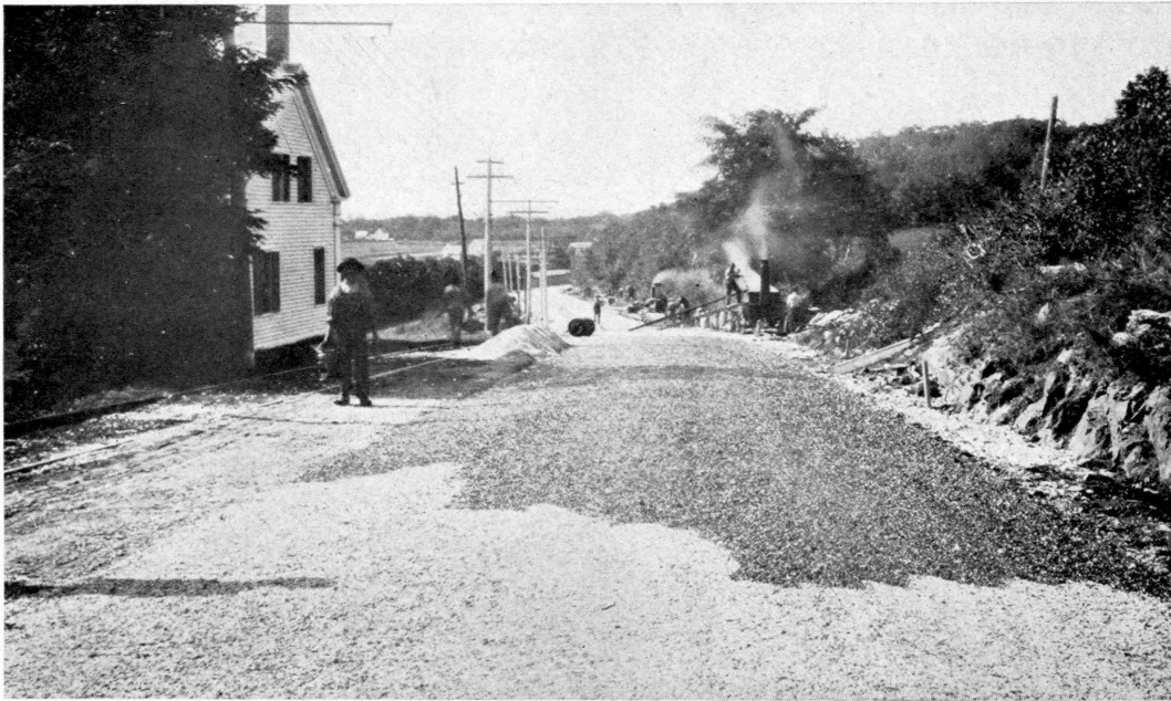
Rockland-Rockport. Trunk Line, showing courses of material and bituminous binder
