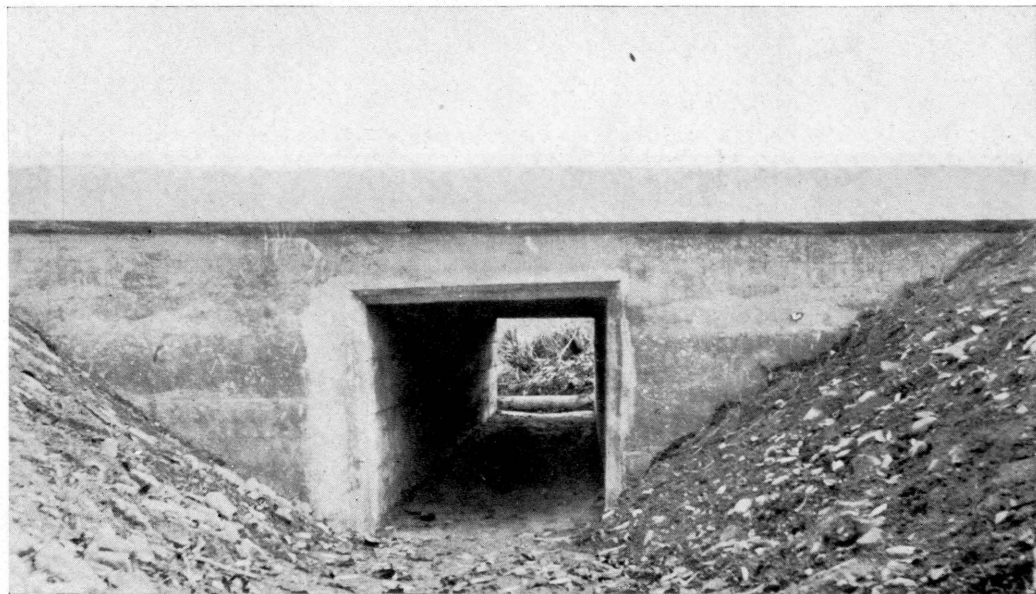
Kittery-Portland. Trunk Line. Reinforced concrete culvert. 1910
