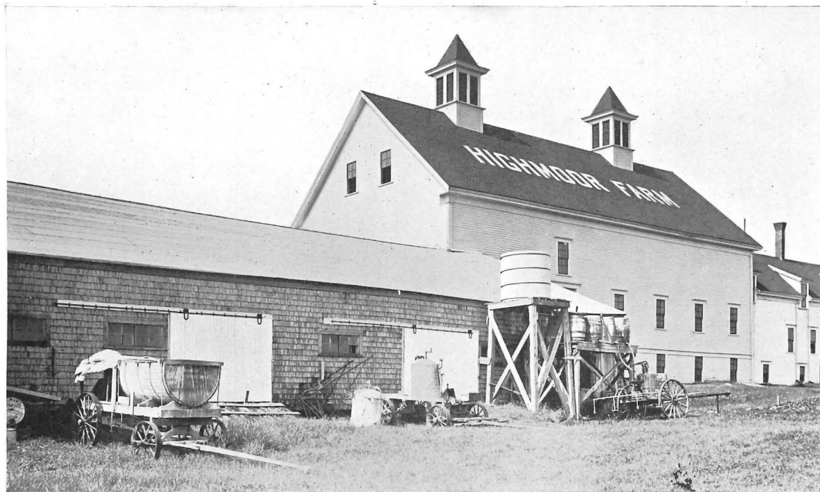
Fig. 83. Elevated platform, at the right, for preparing Bordeaux Mixture. The larger tank on the higher platform is for water storage.
