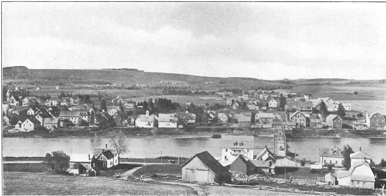
Part of Fort Fairfield village, Aroostook county, Maine.
