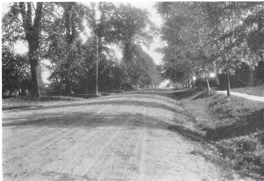
Readfield. 1909 section of State Road. "V" drain foundation; gravel surface.
