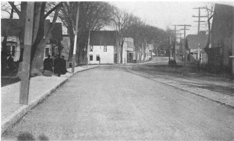
Westbrook. 1909 section of State Road. Bituminous Macadam.
