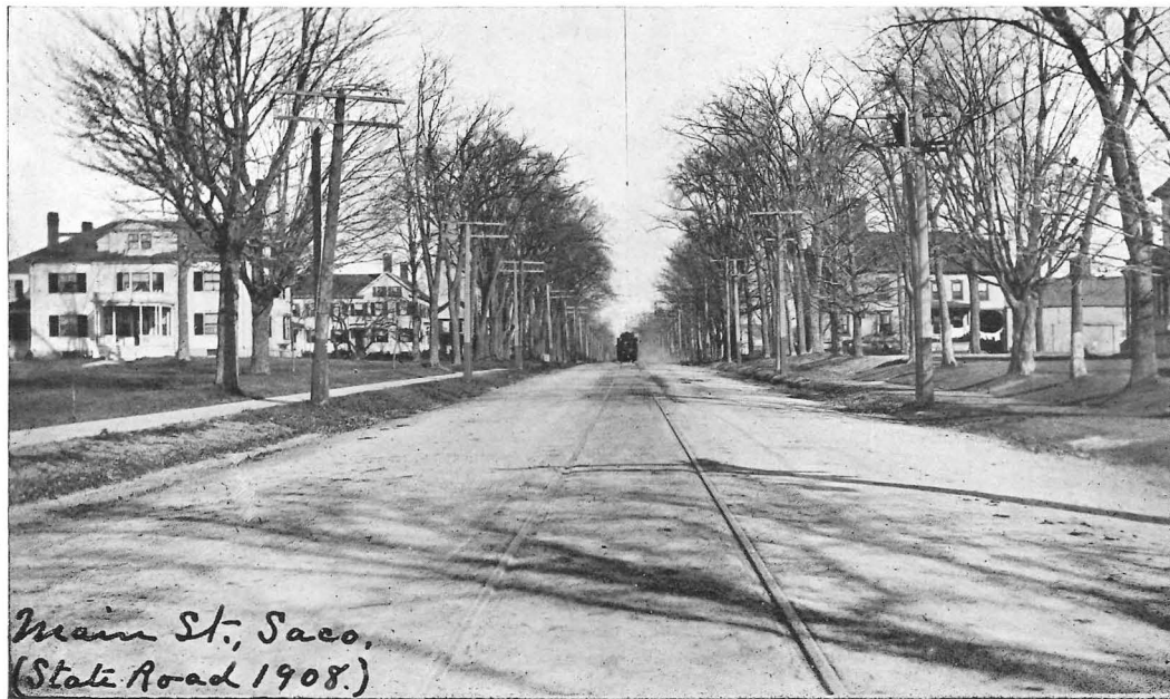
Saco. 1908 section. Macadam, local stone. Contracted to city
