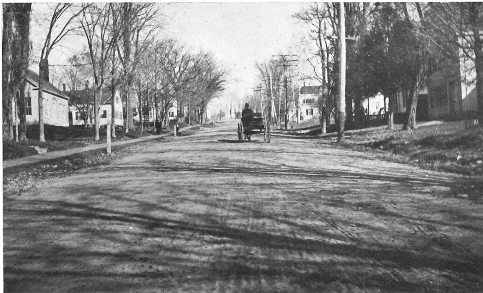
Camden. 1908 section of State road. Finished as per road section "A". Bottom course, run of crusher; top course, selected gravel. Contract let to town. Fred B. Annis, Commissioner
