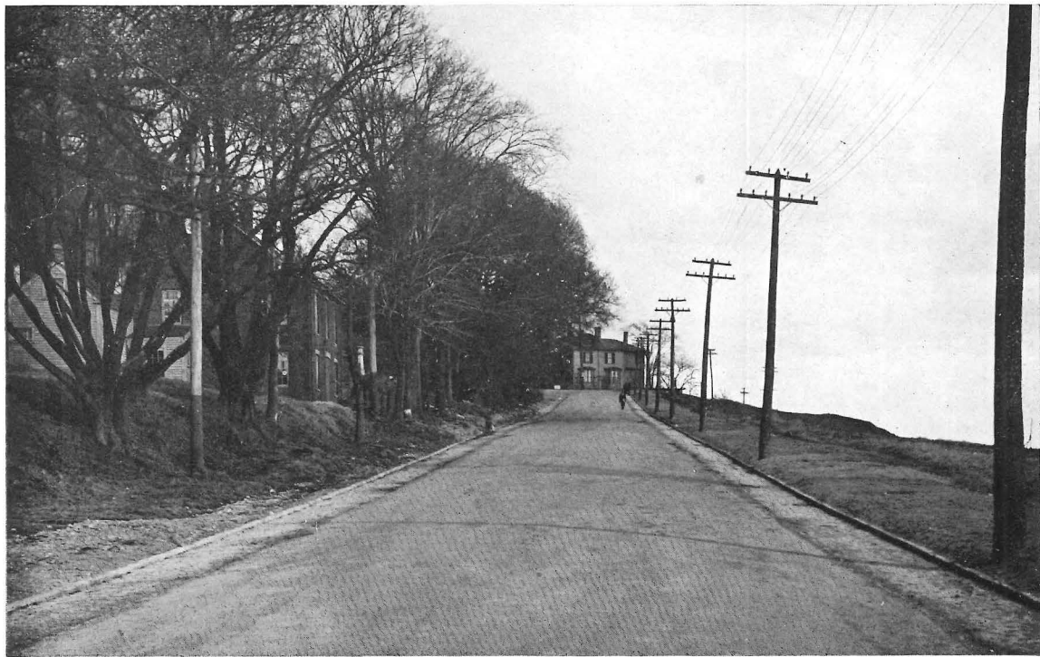
Portland. 1908 section. Finished macadam road, trap rock surface. Contract let to city. Bion Bradbury, Jr., Commissioner of Public Works
