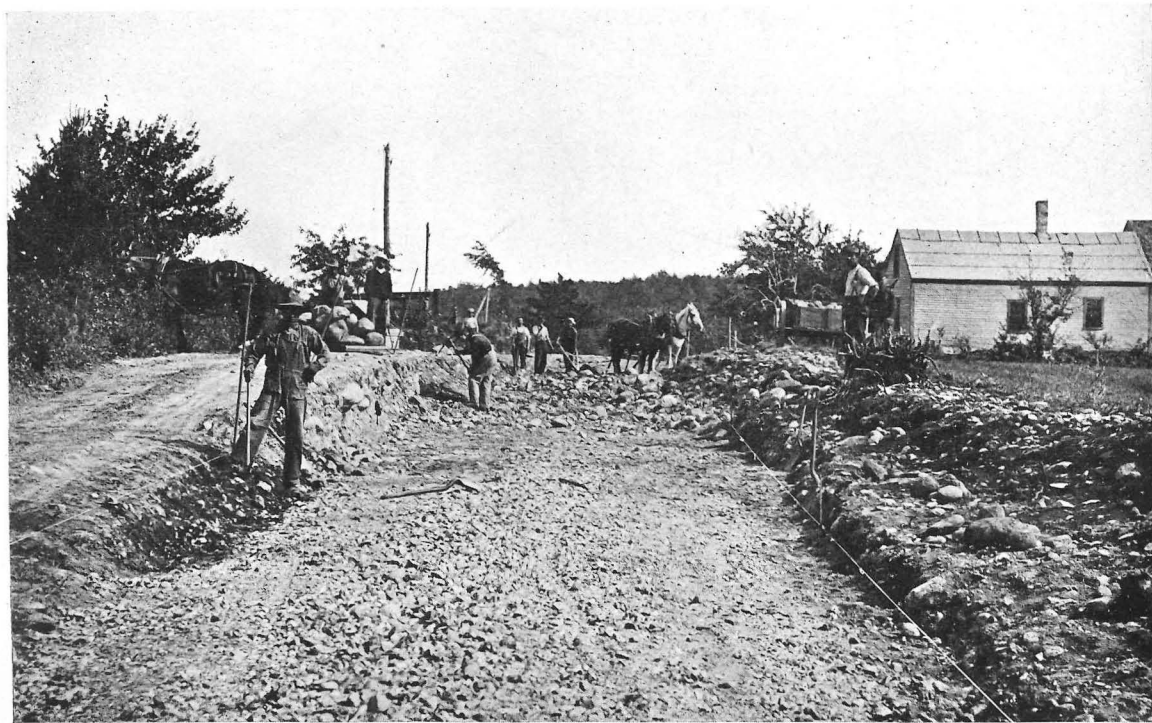
Sanford. 1907 section. Grade reduction. Work done by town. J. G. Ridley, Commissioner
