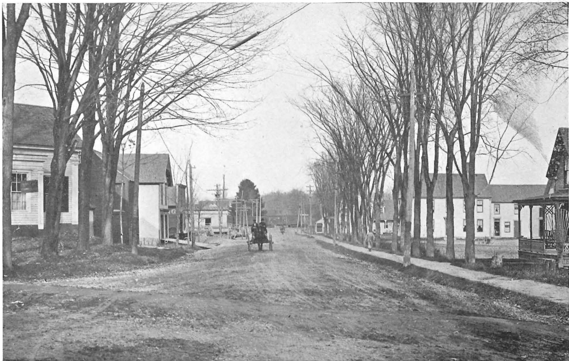
Foxcroft. 1908 section. Macadam, local stone. Built by town. A. A. Adams, Road Commissioner
