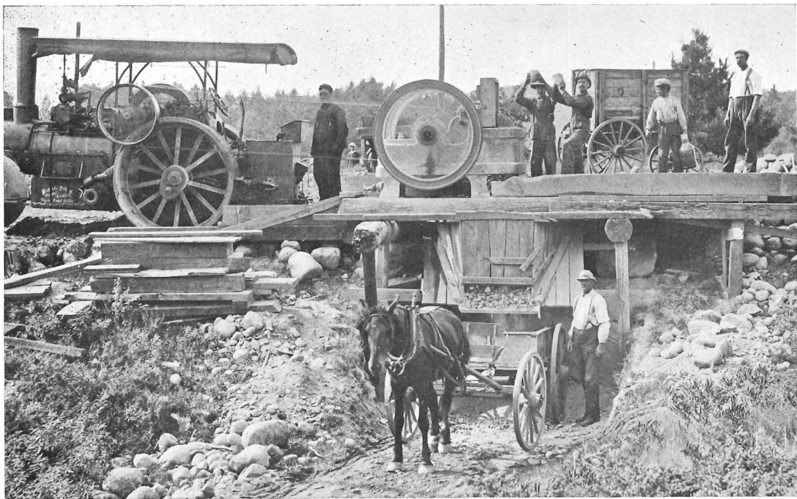
J. G. Ridley, Road Commissioner of Sanford, by this arrangement shows that a rock crusher without elevator and bins may be economically operated
