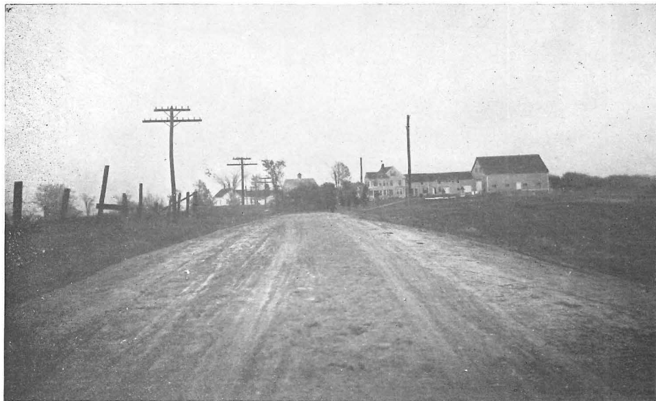
North Yarmouth. 1908 section. Earth surface with "V" drain. Built by town Chas. H. Mitchell, Commissioner
