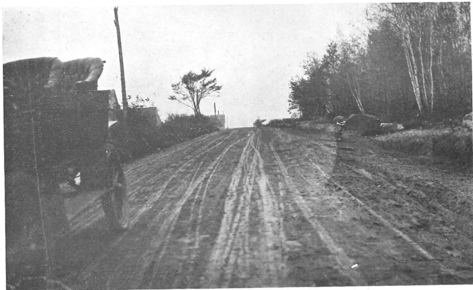
Oakland, 1908 section. Earth surface with "V" drain. Built by town B. J. Libby, Commissioner
