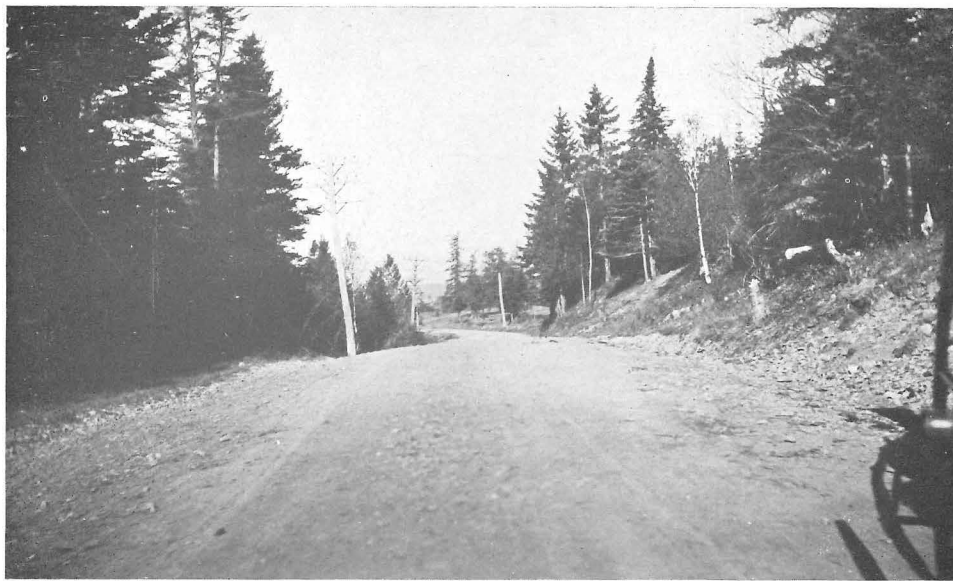
Perry. 1908 section. Gravel road. Built by town. H. F. Hibbard, Commissioner
