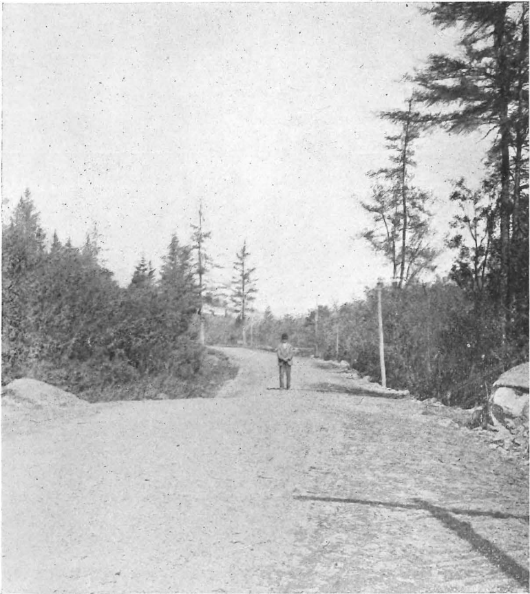
Sorrento. 1908 section after improvement. At this point ledge summit was removed and road widened. Built by town. O. W. Sargent, Commissioner
