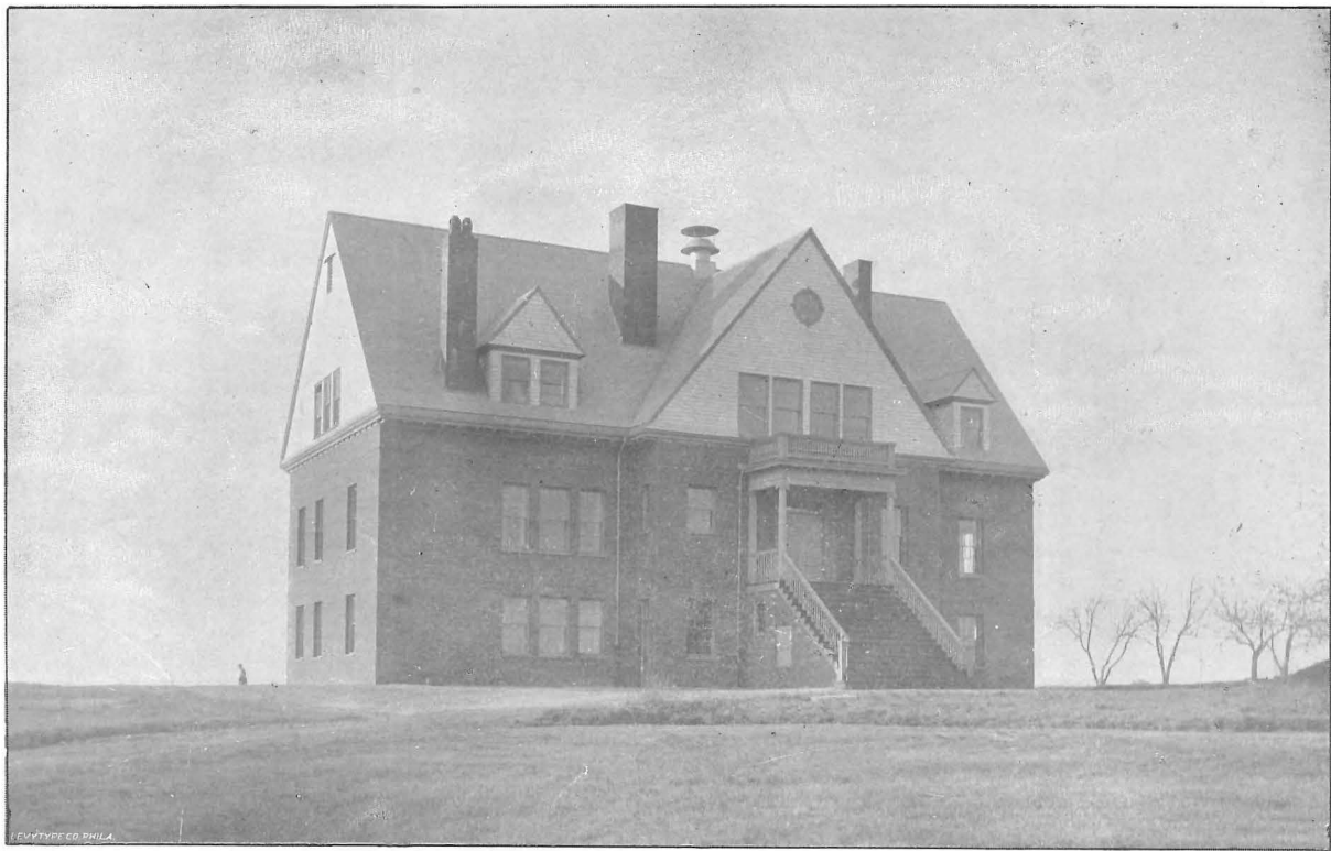
Farrington Cottage, built 1891-92
