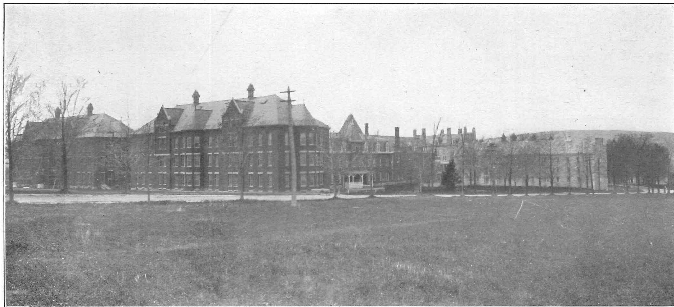
Maine Insane Hospital North View—Female Pavilions and Stone Wings
