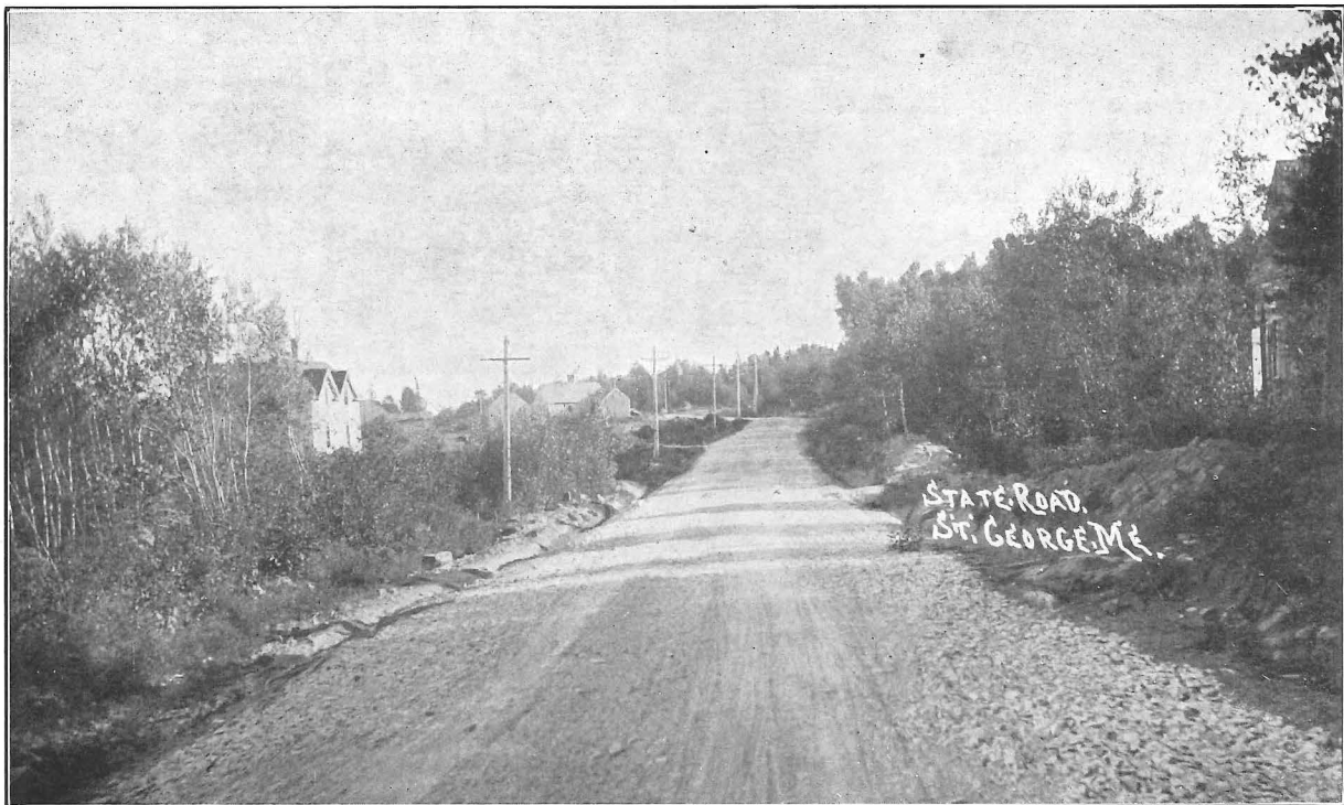
State Road, St. George, Knox County, built 1906 Built from quarry refuse; 18 feet wide, cost 50c per lineal foot. See description in last part of Report
