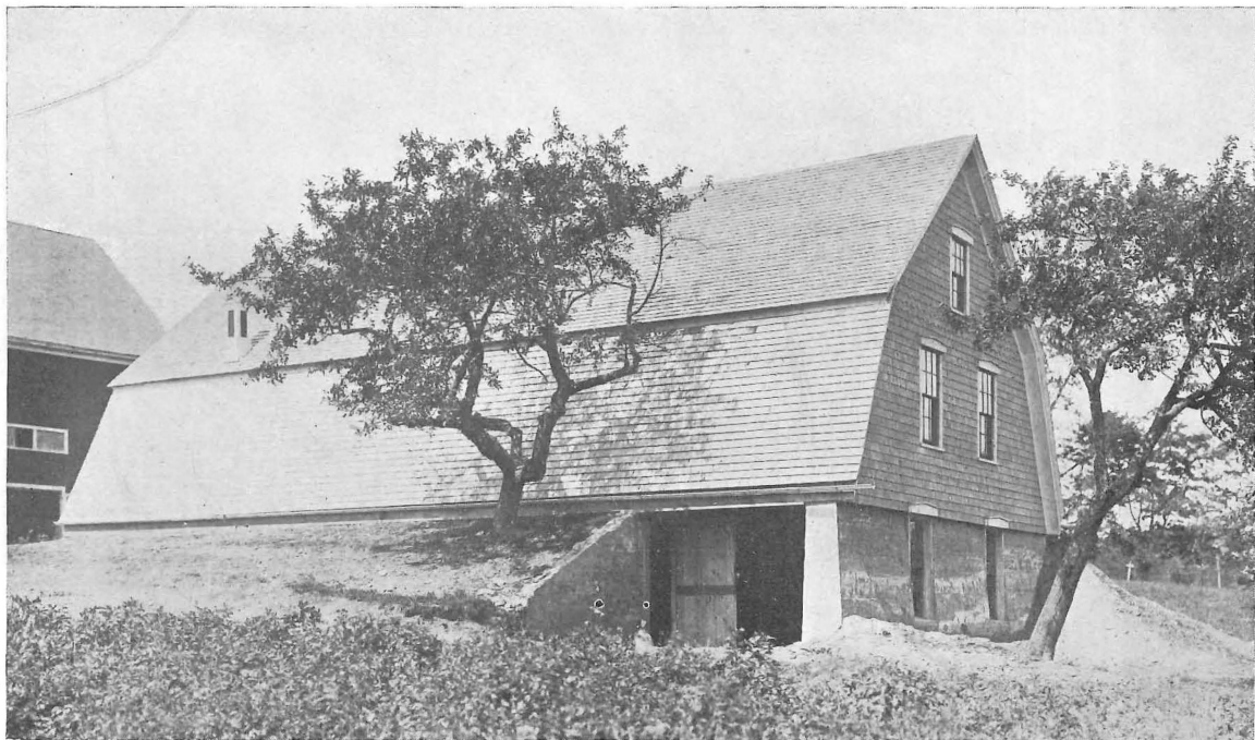
A modern potato cellar. Storage capacity, 6,000 bushels
