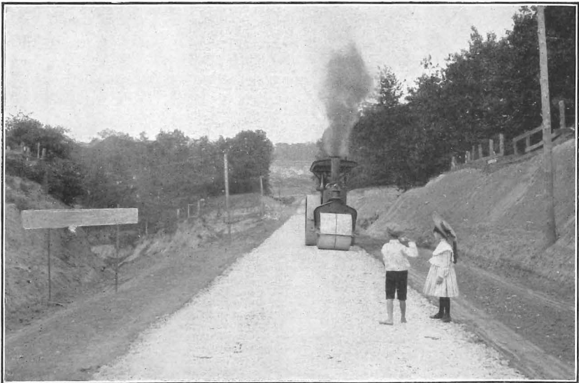
Fig. 2.—The Evolution of a Country Road—4. May 19, 1904. [First course of stone, 4 inches thick, applied; now being rolled.] From Lancaster, Practical Road Building in Madison County, Tennessee, Yearbook, U. S. Department of Agriculture, 1904.
