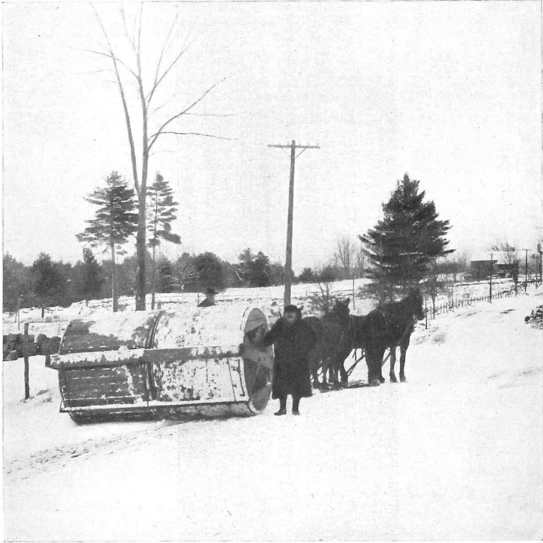
Equipment used in Town of Bridgton for making Winter Roads. Town owns 12 of these rollers which are kept at different points. Cost of rollers, $50.00 each. Cost of rolling roads reported to average 50 cents per mile for each storm.
