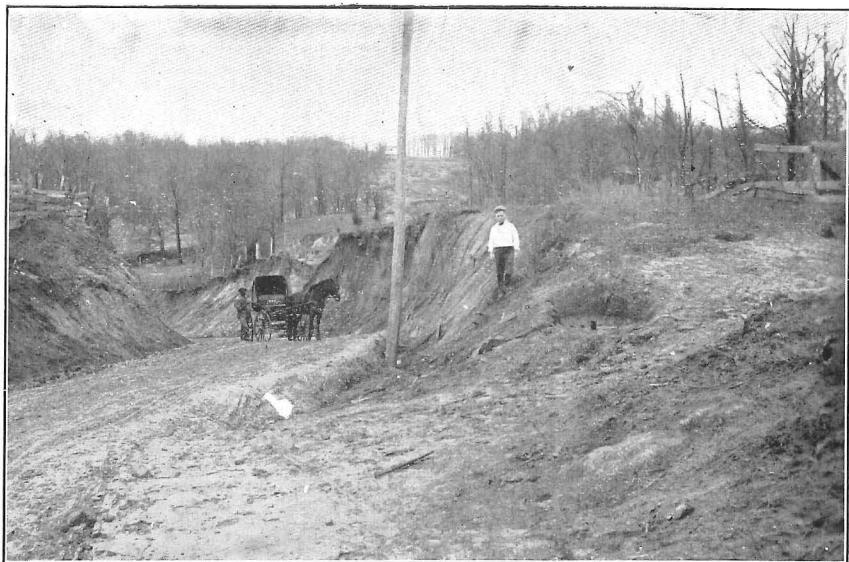
Fig. 1.—The Evolution of a Country Road—1. April 15, 1904. [At this point the road was straightened and placed on better ground.] From Lancaster, Practical Road Building in Madison County, Tennessee, Yearbook, U. S. Dept. of Agriculture, 1904.
