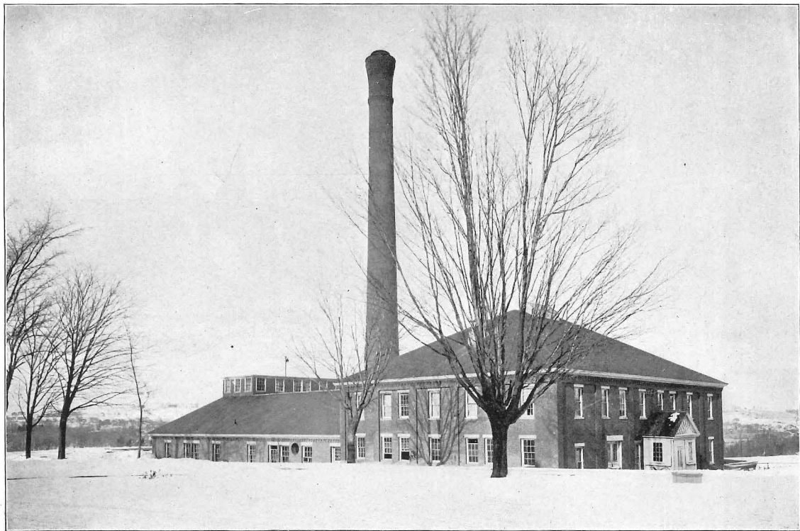
LAUNDRY, POWER HOUSE AND COAL POCKET.
