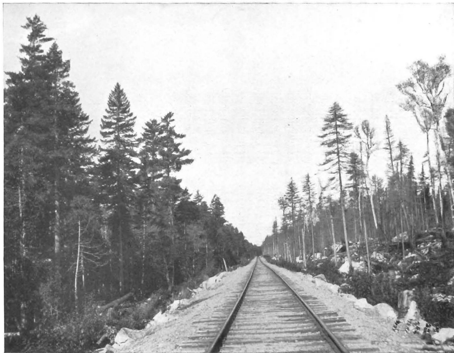
A situation where the right-of-way proved an effective fire-line. Near Bemis, Franklin Co.
