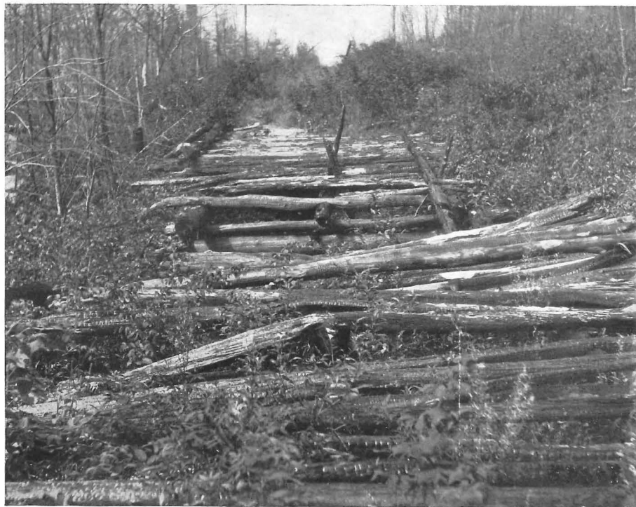
A corduroy road after the 1903 fire. Near Summit, Franklin Co,
