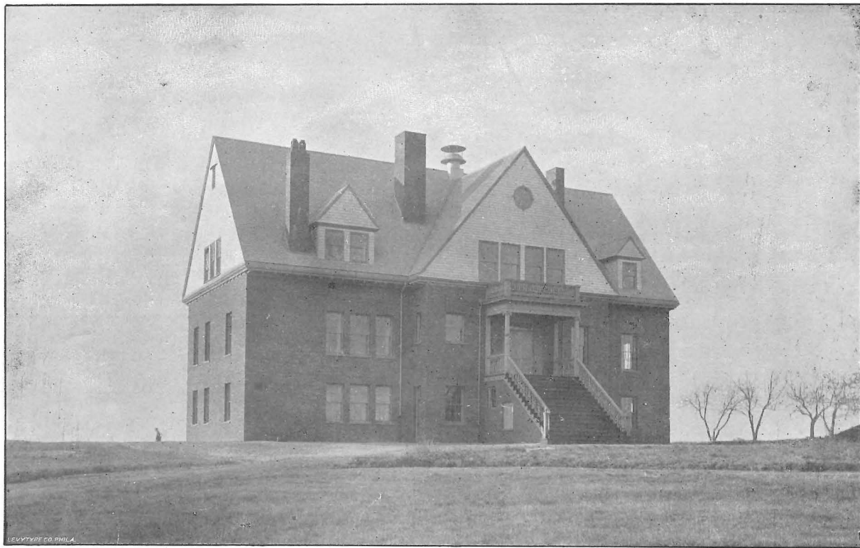
COTTAGE AT STATE SCHOOL FOR BOYS, BUILT 1891-92.
