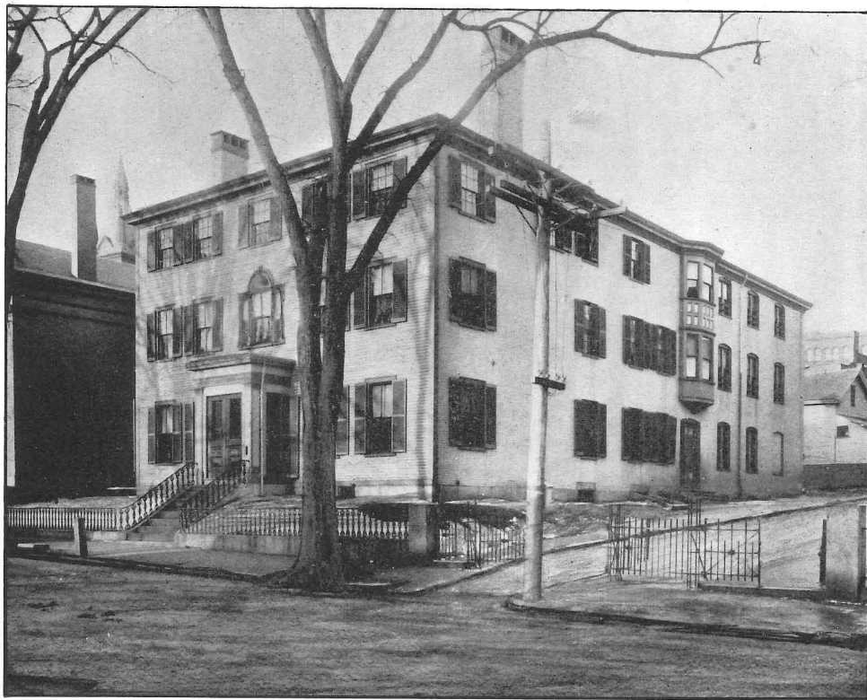
BROWNSON HALL—BOY'S DORMITORY.
