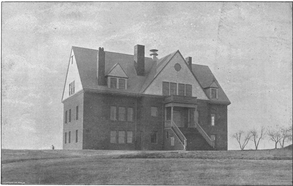
COTTAGE AT REFORM SCHOOL, BUILT 1891-92.
