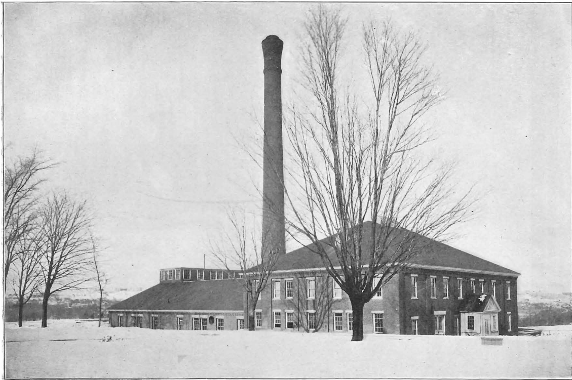
LAUNDRY, POWER HOUSE AND COAL POCKET.
