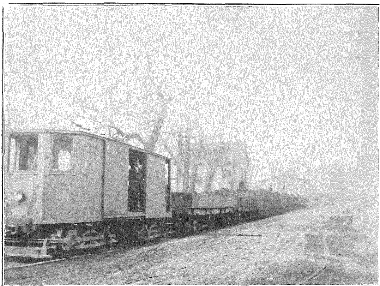
TWENTY-TON ELECTRIC FREIGHT MOTOR HAULING 100 TONS OF COAL. SANFORD AND CAPE PORPOISE RAILWAY.
