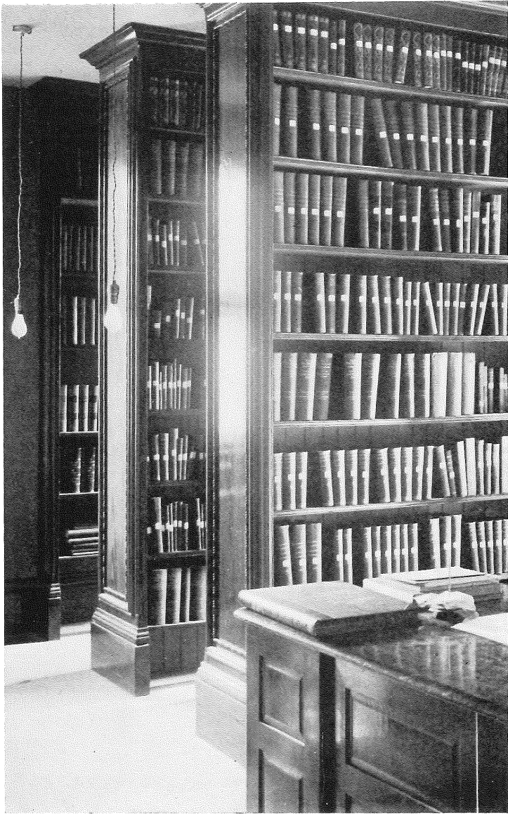
STACK ROOM—CUMSTON HALL.
