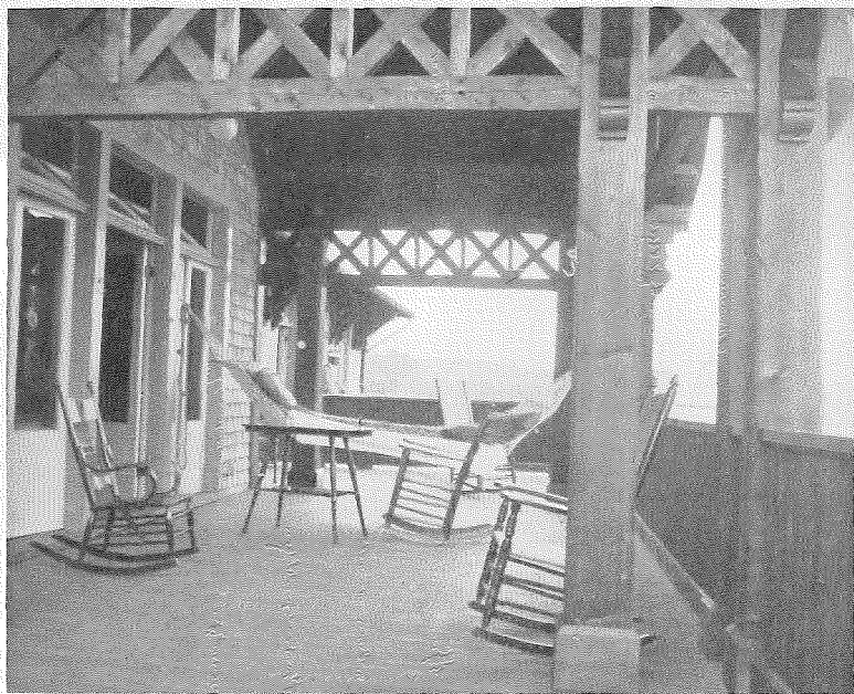
FIG. 30. Loomis Sanitarium—Balcony, Second Floor of Cottage.
