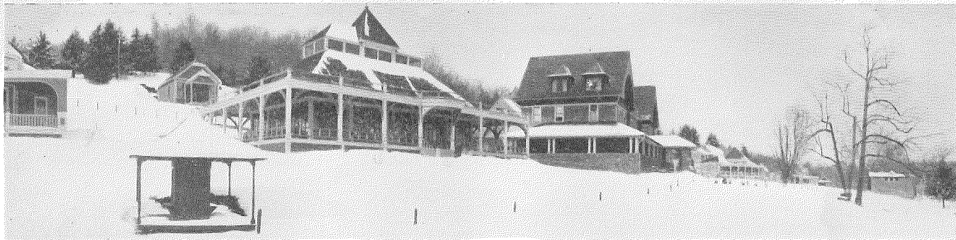
Fig. 15. Adirondack Cottage Sanitarium—Recreation Pavilion, Main Building, and Cottages.
