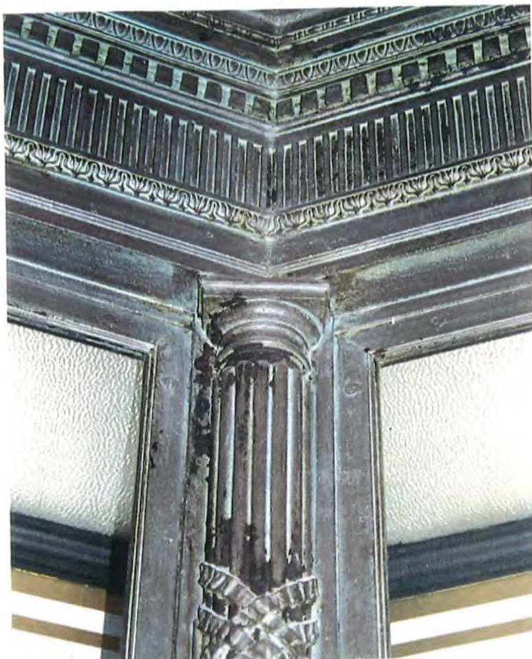
12. Detail of Hall of Flags Cases deterioration
