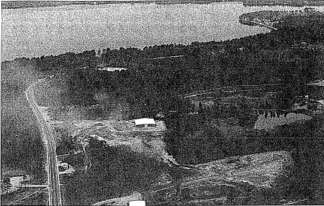
■ THIS landfill once had an incinerator on-site and the ash was buried. A synthetic cap will be installed.
