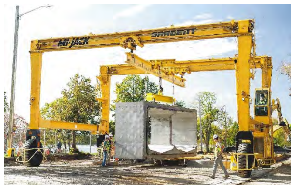
Shawn Newton sets the precast boxes on the Back Cove Storage Conduit project.
