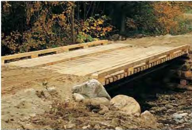
A permanent bridge.
