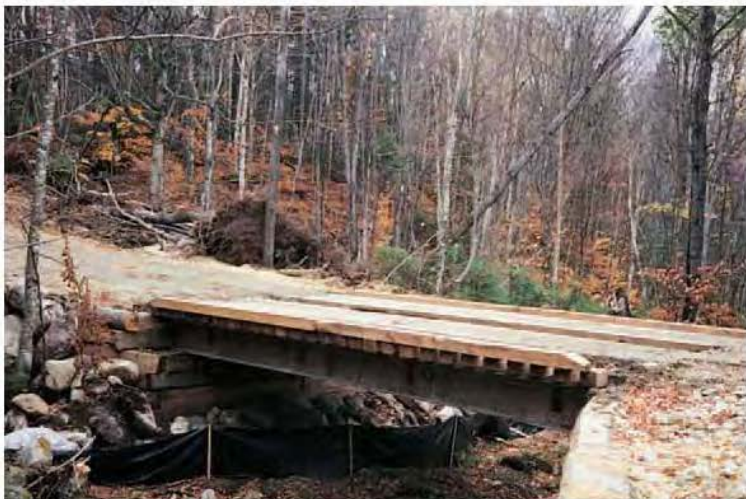
A permanent bridge on a truck road.
