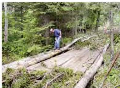
A temporary bridge.
