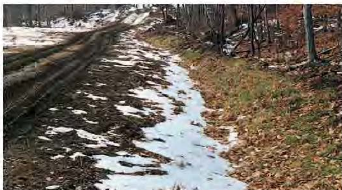
Revegetated road ditches carry water without eroding.
