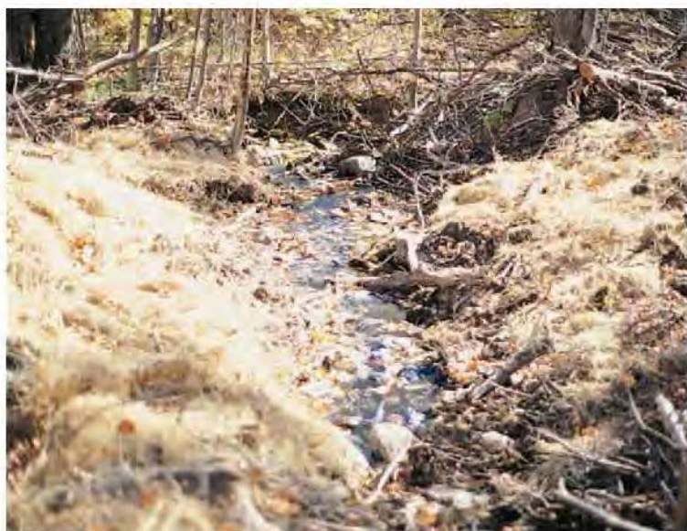
Closeout of a temporary stream crossing.
