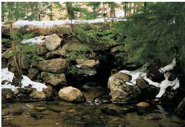
An old stone culvert still functioning.
