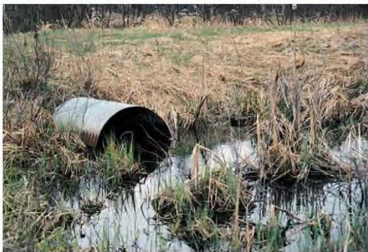
Wetland culverts allow for cross drainage if the road fill does not.
