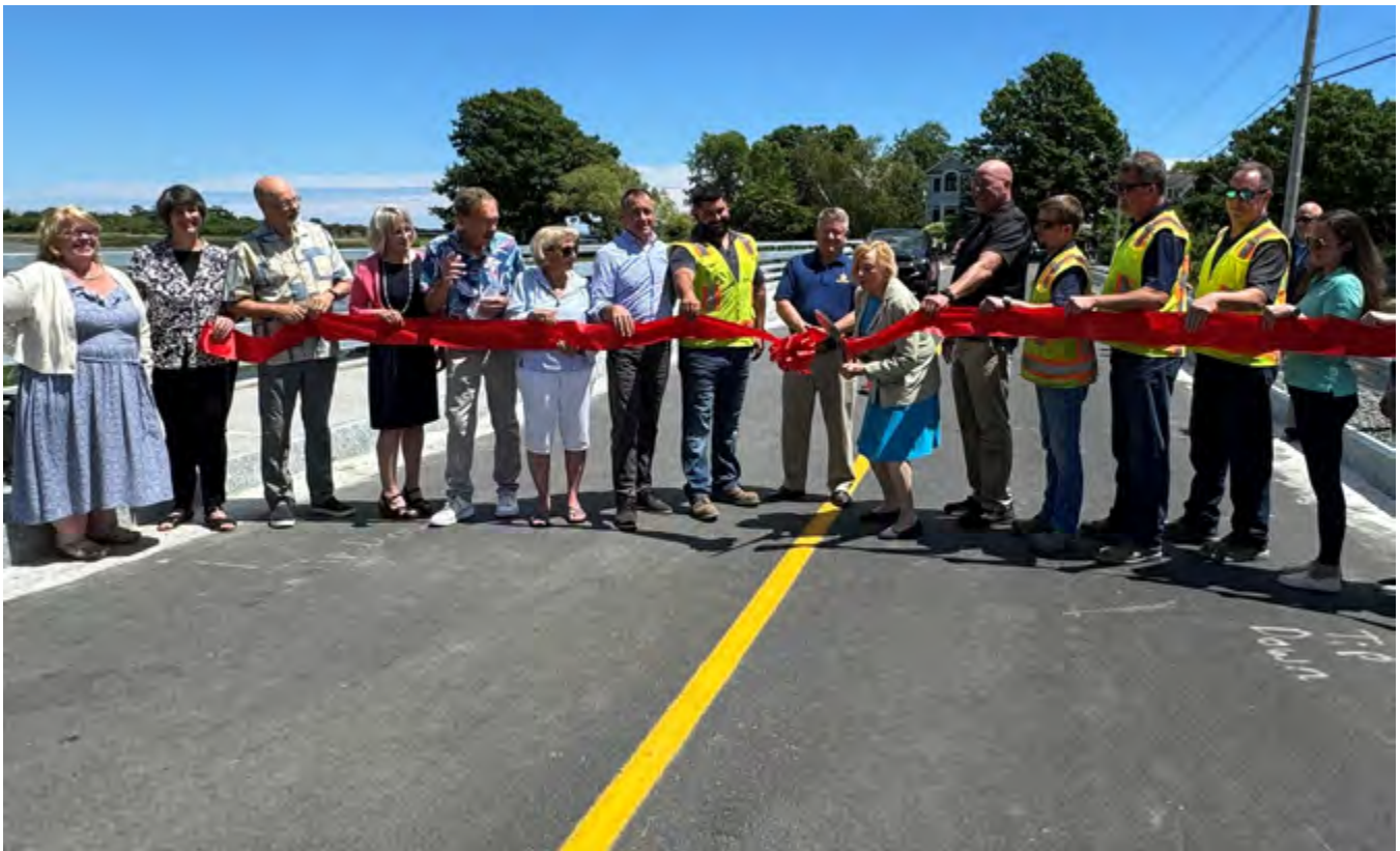
Governor Mills cuts a ribbon re-opening the Pier Road Causeway in Kennebunkport on July 1, 2024, after it was raised 4 feet higher to protect access and infrastructure. The project was made possible with funds from the Maine Infrastructure Adaptation Fund.
