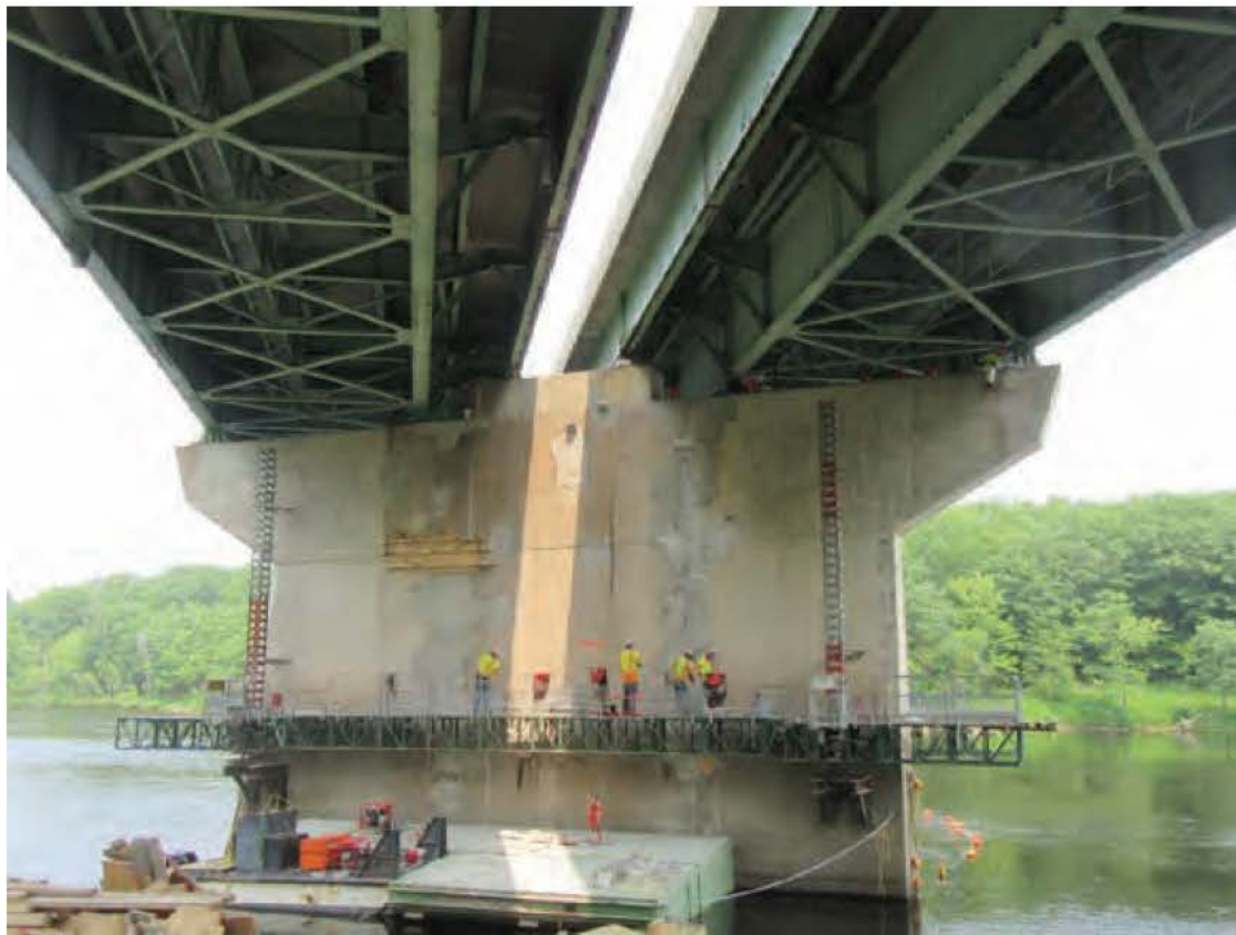
Androscoggin River Bridge Pier Rehabilitation, July 2019.
