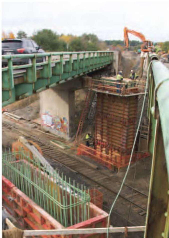
New piers will support a wider bridge over the Maine Central Railroad in Falmouth.
