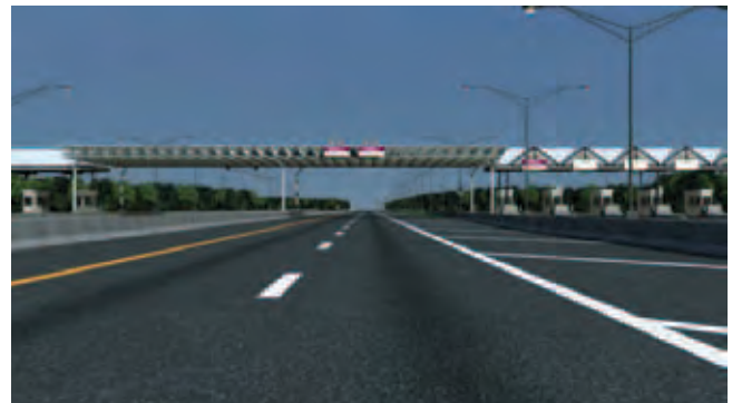
With open road tolling, E-ZPass customers will pay tolls at normal highway speeds by passing beneath a canopy with sensors (photo simulation).
