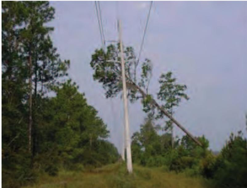
**Figure 3-1.** Tree falling into transmission lines.
