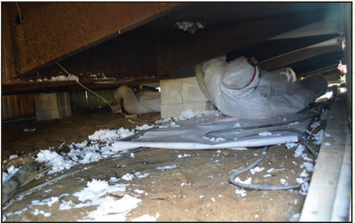
2016: Workers blow in insulation under a Scarborough mobile home as part of a full-house weatherization service by The Opportunity Alliance and MaineHousing.
