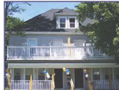
44 Fairfield Street in Oakland, providing 6 units of housing to people who were homeless.
