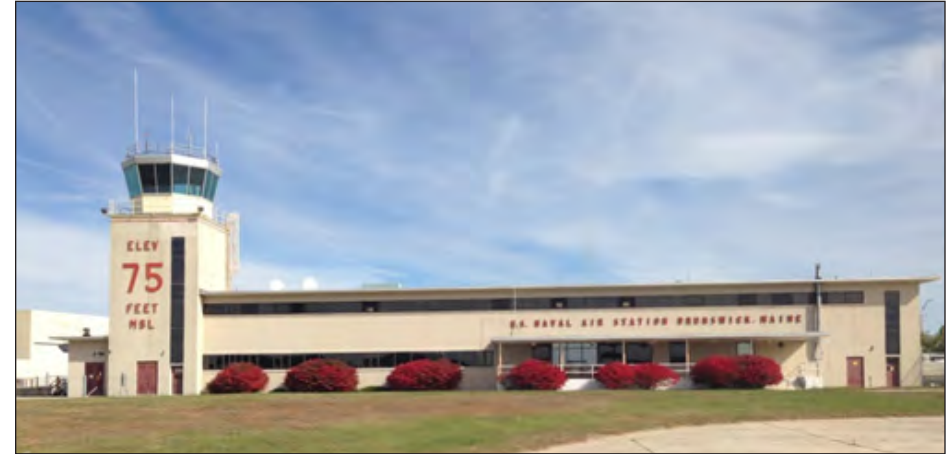
The former Navy Air Operations Building is being converted into an air terminal with grant funds from the FAA's Military Airports Program.
