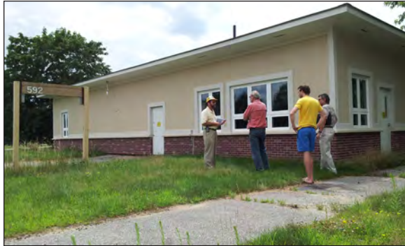
Larry Carbury of Dow Corning debriefs building owner Tom Wright on the energy-efficiency improvements made to former Navy Building 592 after a one-year study.
