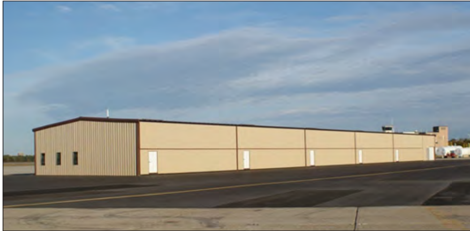
New 10-Unit T-Hangar provides aircraft storage for airport tenants. It opened in August and already hosts eight airplanes.
