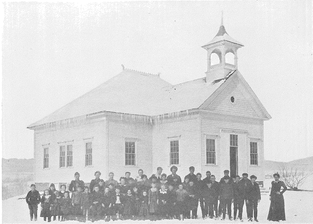
FAIRBANKS SCHOOL BUILDING, FARMINGTON.
