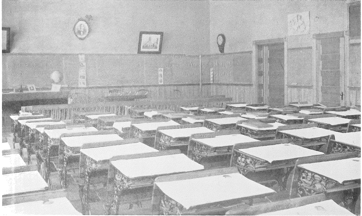
CLASSROOM, PARKER SPOFFORD GRAMMAR SCHOOL BUILDING.
