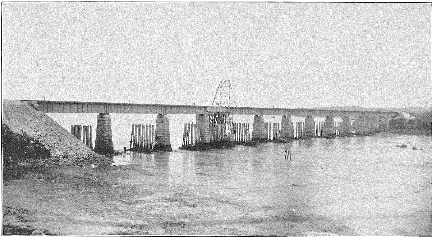
NO. 1. THE NEW STEEL GIRDER, On the Maine Central Railroad at Thomaston, replacing the wooden bridge.
