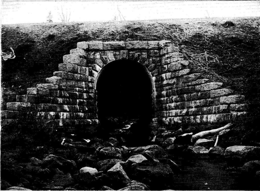
ARCH CULVERT. SLATE ROCK WITH GRANITE END COURSES; C. P. RAILWAY NEAR LOWELLTOWN.
