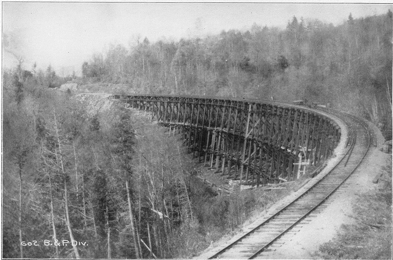
BUNKER TRESTLE; PISCATAQUIS DIVISION, BANGOR & AROOSTOOK RAILROAD.
